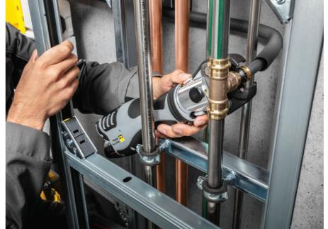
The Pressgun Picco 6 Plus excels when space is limited and enables single-handed pressing in any situation.
