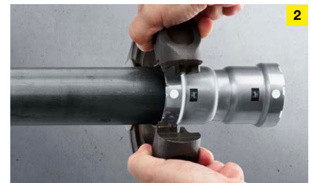
For pressing Megapress S connectors from 1 ¼ inch upwards, only press rings with hinged adapter jaws are used. For smaller sizes between ½ and 1 inch, both press jaws and press rings with hinged adapter jaws are available.
