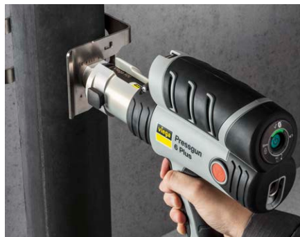
Press the press-in branch connector in the pipe with the pressgun insert.
