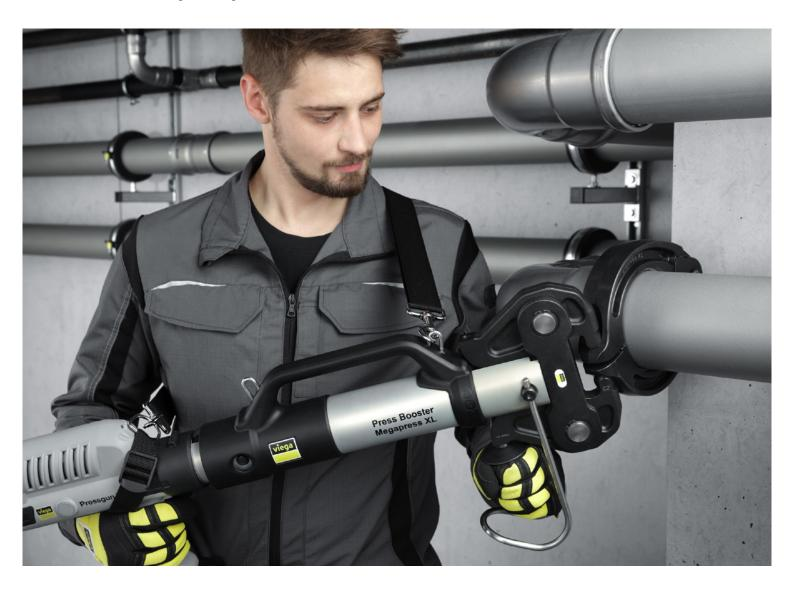
Viega's launch of the industry-first Megapress system allowed thick-walled steel tube to be press connected for the first-time, making installation fast, safe and simple. Since then, Viega has constantly pushed the technology forward and press connections can now be used on tube up to four inches in diameter - providing an alternative to welded, threaded and grooved connections.
