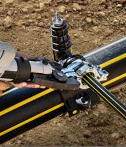
Using Press Gun to close the connection.
