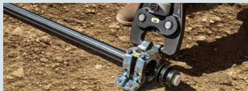
3. Press the connector and check the green pressing marker.
