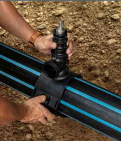
Applying the tapping valve.
