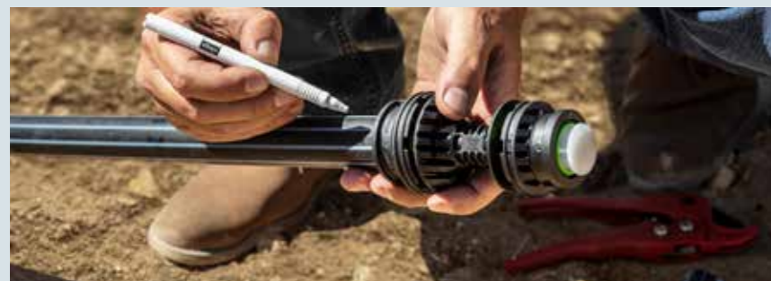
2. Place connector onto pipe. Check the insertion depth in the window and draw a safety mark on the pipe.
