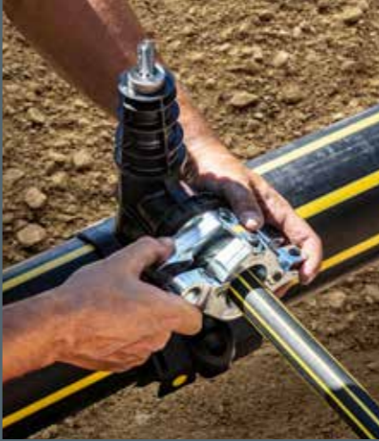
Positioning coupling.
