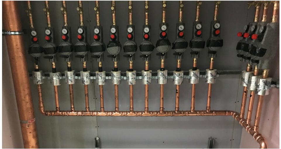
Viega's copper Profipress system was used extensively with a size range from 12 to 108mm.
