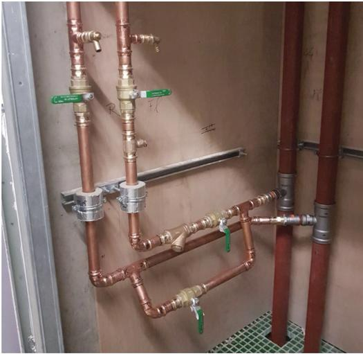
The installation team could easily switch between pressing copper and steel by changing tooling in Viega's Pressgun 5 machine.
