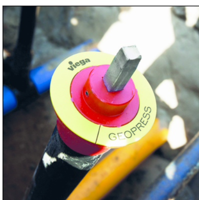
Fig. 6: Marking – gas = yellow
